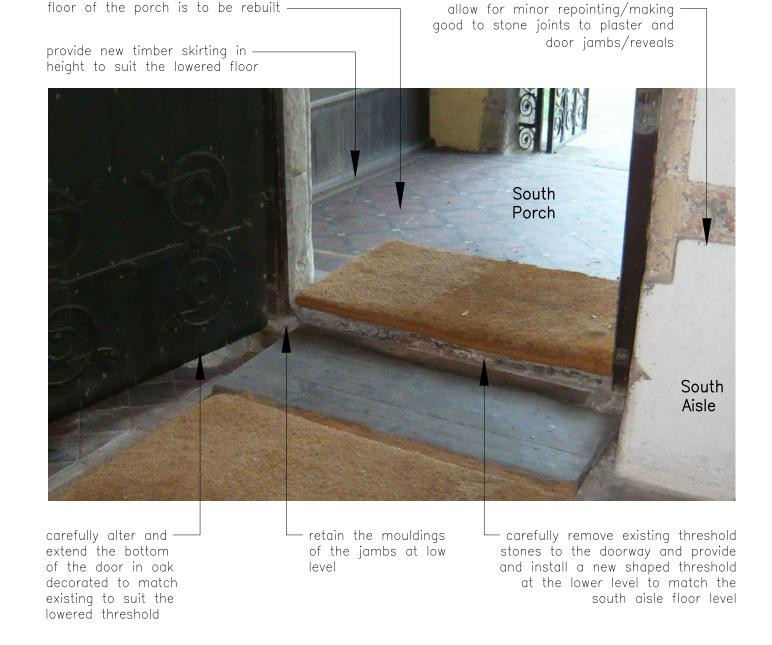
The floor of the porch is to be rebuilt so that it is level with the outside of the new threshold under the door into the south aisle. The new porch floor level will be 25mm above the south aisle floor level.
